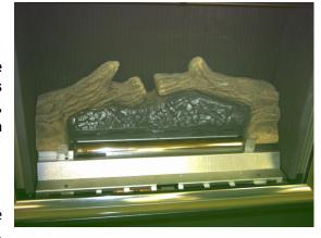
8.1.1 Carefully place the rear (largest) log piece on the support platform behind the burner.
