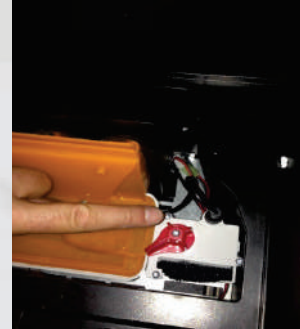
3. Check wires are still secure
