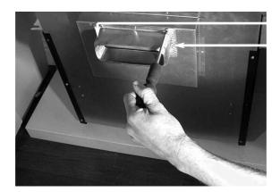
4 off Flue Spigot Fixing screws
