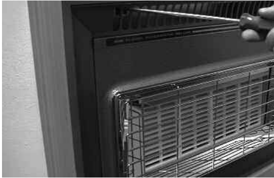
Fig. 10 Removing the Upper Outer Case Fixing Screws
