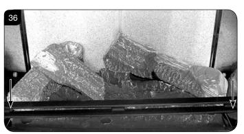
7.23 Place Log A across Log C. There is a hole on the underside of Log A which fits over the raised stud on Log C to secure in place. The small cut out on the left side of the log rests onto the log guard, see Diagram 37.
