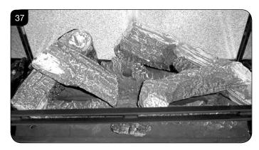
7.24 Once the logs are in place use some of the Embaglow wire wool provided and cover the ports in the burner tray with a liberal amount of fibres, in the highlighted areas shown in Diagram 38.
