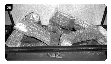
8.24 Once the logs are in place use some of the Embaglow wire wool provided and cover the ports in the burner tray with a liberal amount of fibres, in the highlighted areas shown in Diagram 29.
