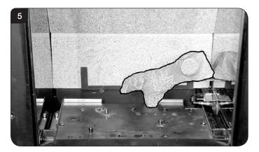
7.4 Place Log B over the two middle studs on the burner tray, see Diagram 6.
