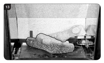
6.4 Place Log E onto the stud and behind the tag on the left hand side of the burner tray. Rest against Log B, see Diagram 14.
