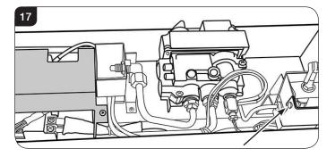
8.2 Cut the cable tie retaining the vida flex sleeve and disconnect the ignition lead from the electrode.
