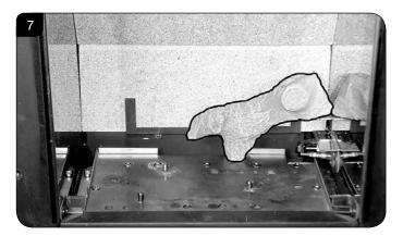
7.3 Place Log B over the two middle studs on the burner tray, see Diagram 8.
