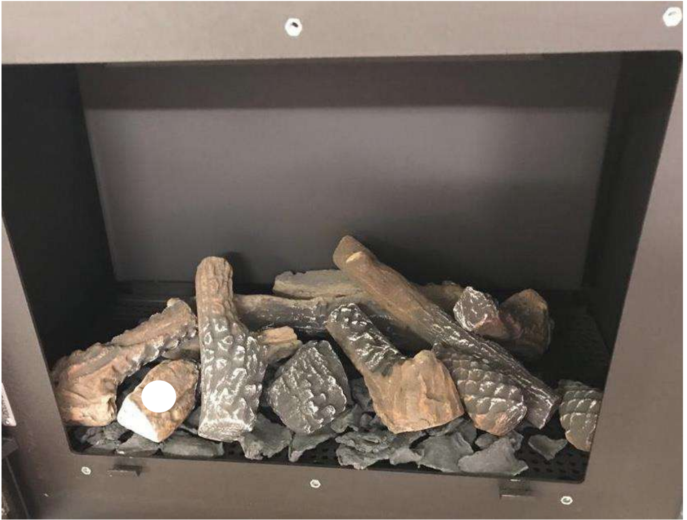
Step 11 - Position Ceramic Log 7 (1st one) so it sits at the front – as per the picture above – As marked with the White Dot
