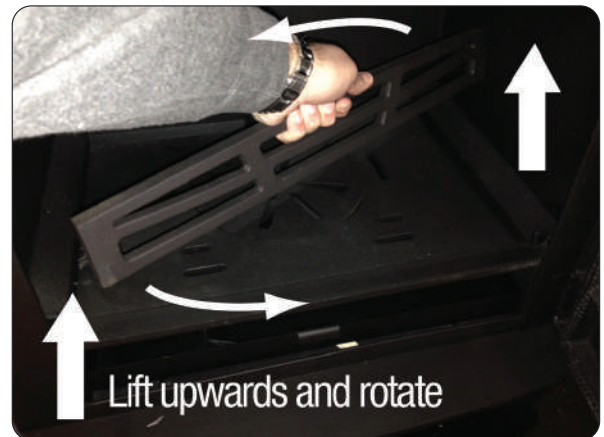
Lift Retainer Upwards & Rotate
